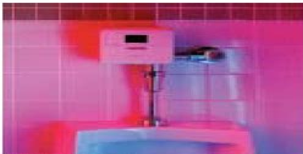
Fig. 1: Installation of the automatic flush system
