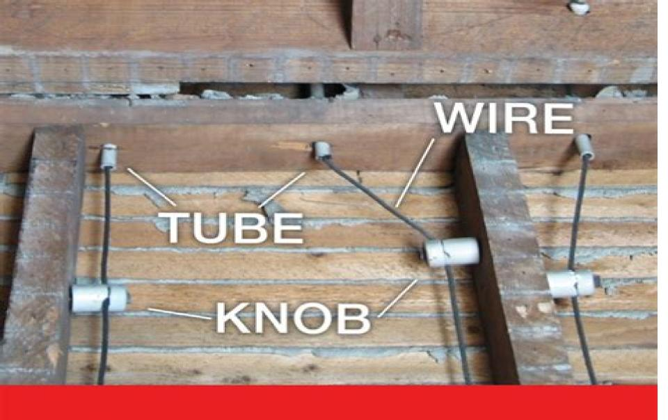
KNOB AND TUBE WIRING
