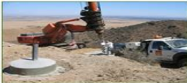
Foundation construction for an LST.
