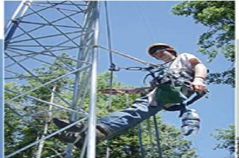
Left: The height of the towers compounds the dangers of installing and maintaining wind turbines. Above: Zander Woofenden demonstrates leaning out in a working position. Note that he is still clipped into the safety cable.
