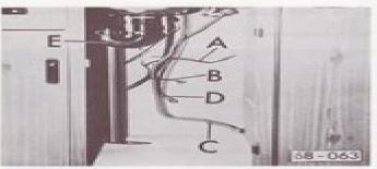
remove fuse in in-line fuse holder for water pump, disconnect hot wire (A) and ground wire (B) from fuse box, gas range connection (C) and city water hook-up (D) (E = sink drain pipe)
